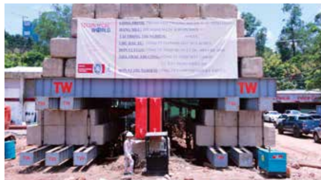
Kentledge System with the capacity up to 6000 Tons
