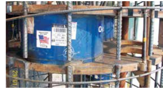
Pile load test by Osterberg (O-Cell) method
