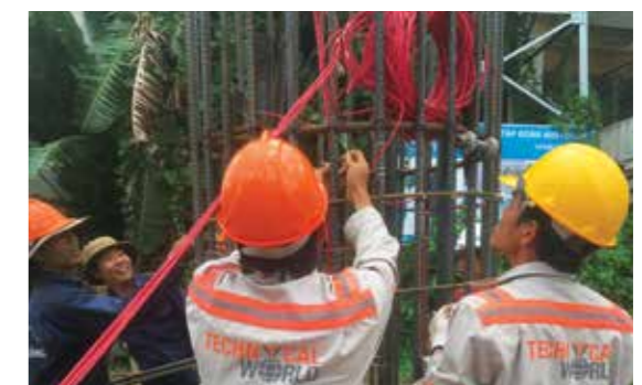
Pile body shortening measurement
