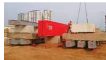
Prop-beam and main beam installation
