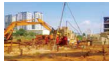
Anchor pile construction
