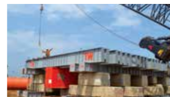
Independent girder & turnbuckle installation
