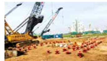
Anchor head covering installation
