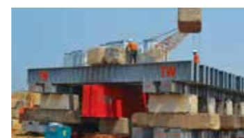
Load concrete blocks to the system
